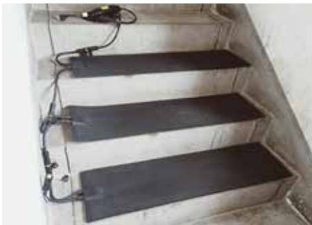
Ice melting for stairways
